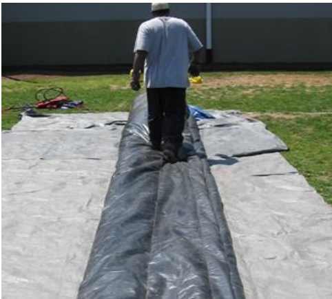
Fold one half over the other half. Walk out air toward ports.
